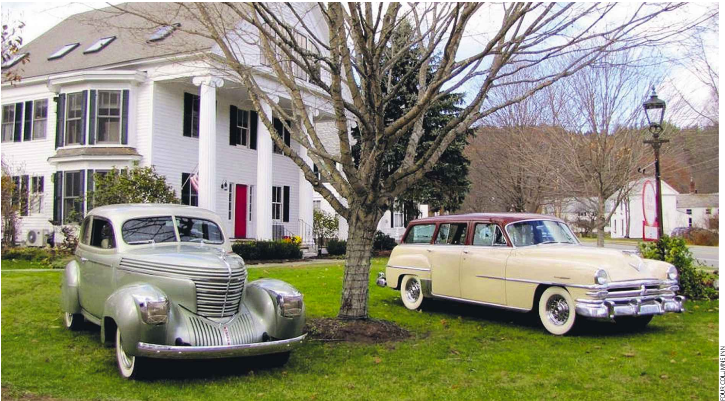
The Four Columns Inn in Newfane, Vermont, went through a major renovation a few years ago.
